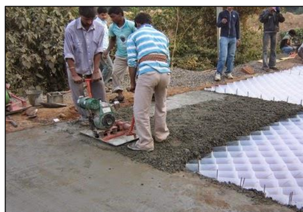
Figure 60 Laying of Cell filled Concrete Pavement.
