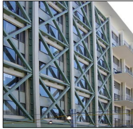
Figure 56 Infill Shear Truss
