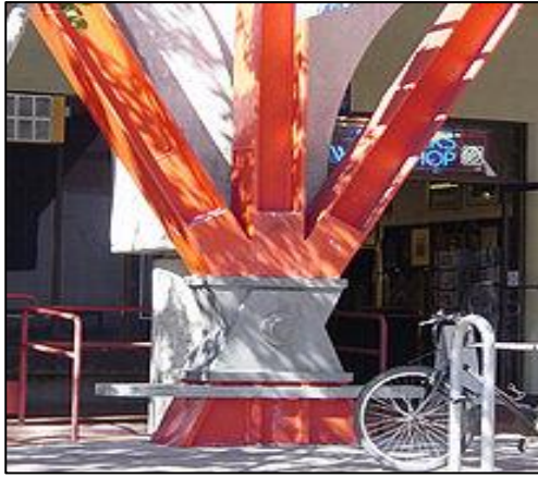
Figure 55 External Bracing of an Existing Structure
